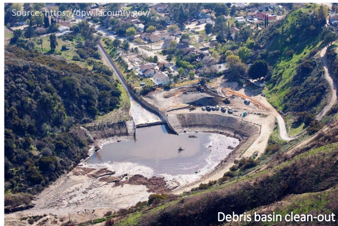
Below: Example of debris basin clean-out
