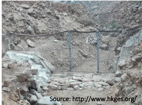
Left: Installation of large boulders (i.e., riprap) to reinforce debris fence anchor base; Right: Picture of exposed debris fence foundation that no longer is protected by riprap after a flood event.
