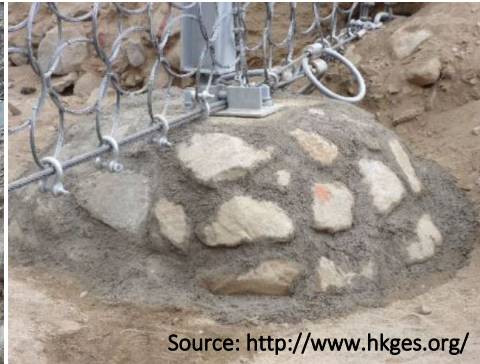
Left: Installation of large boulders (i.e., riprap) to reinforce debris fence anchor base; Right: Picture of exposed debris fence foundation that no longer is protected by riprap after a flood event.
