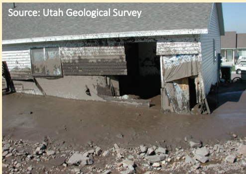
Above: Wall breached by force of debris flow
