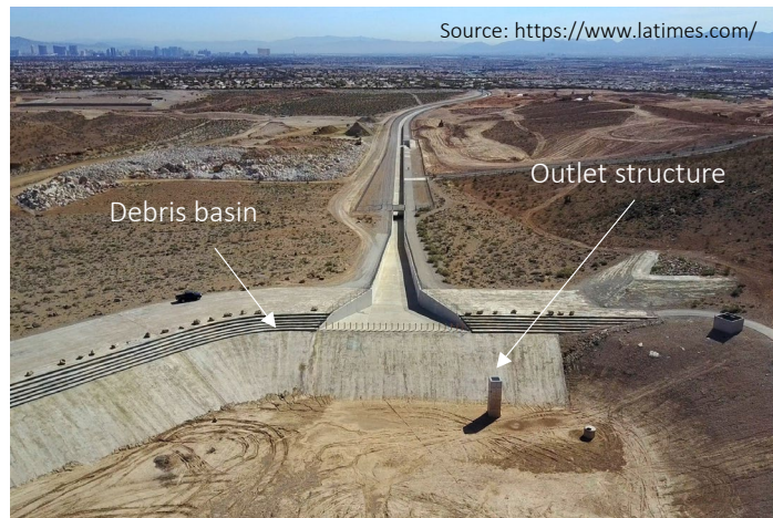
Above: Example of debris basin with outlet structure
